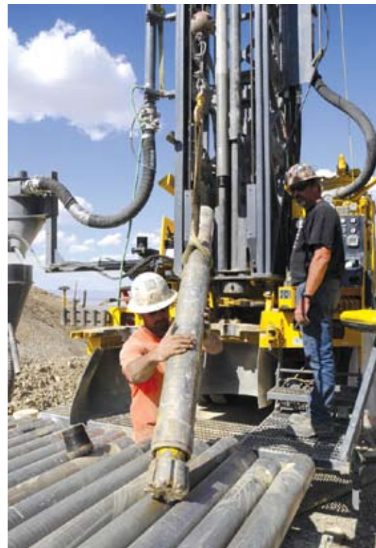
Hoisting the RC50 DTH hammer in place.
