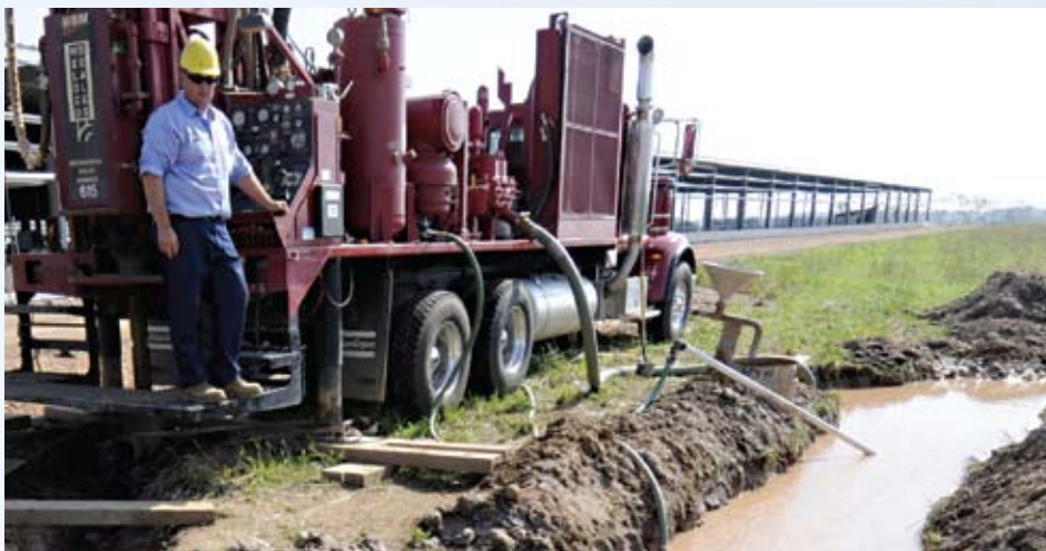
Behind Jeff Haughian you can see the 1,000 ft (305 m) long dairy barn which he is drilling a 100 gpm (455 lpm) well that will be used for a cow cooling system. They are mud drilling the first 240 ft (73 m).
