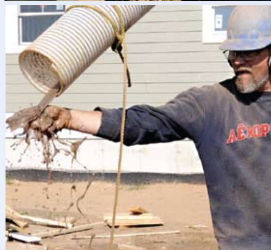
Behind Jeff Haughian you can see the 1,000 ft (305 m) long dairy barn which he is drilling a 100 gpm (455 lpm) well that will be used for a cow cooling system. They are mud drilling the first 240 ft (73 m).
