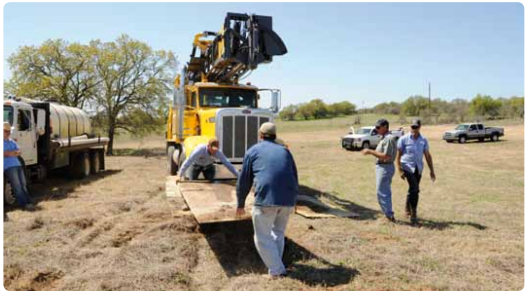
Taylor Virdell seals the casing with bentonite. Heavy rains have made it difficult to reach some drill locations. Without portable fiberglass mats the rig buried to the axles.
