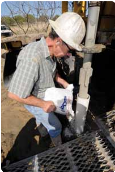
Taylor Virdell seals the casing with bentonite. Heavy rains have made it difficult to reach some drill locations. Without portable fiberglass mats the rig buried to the axles.
