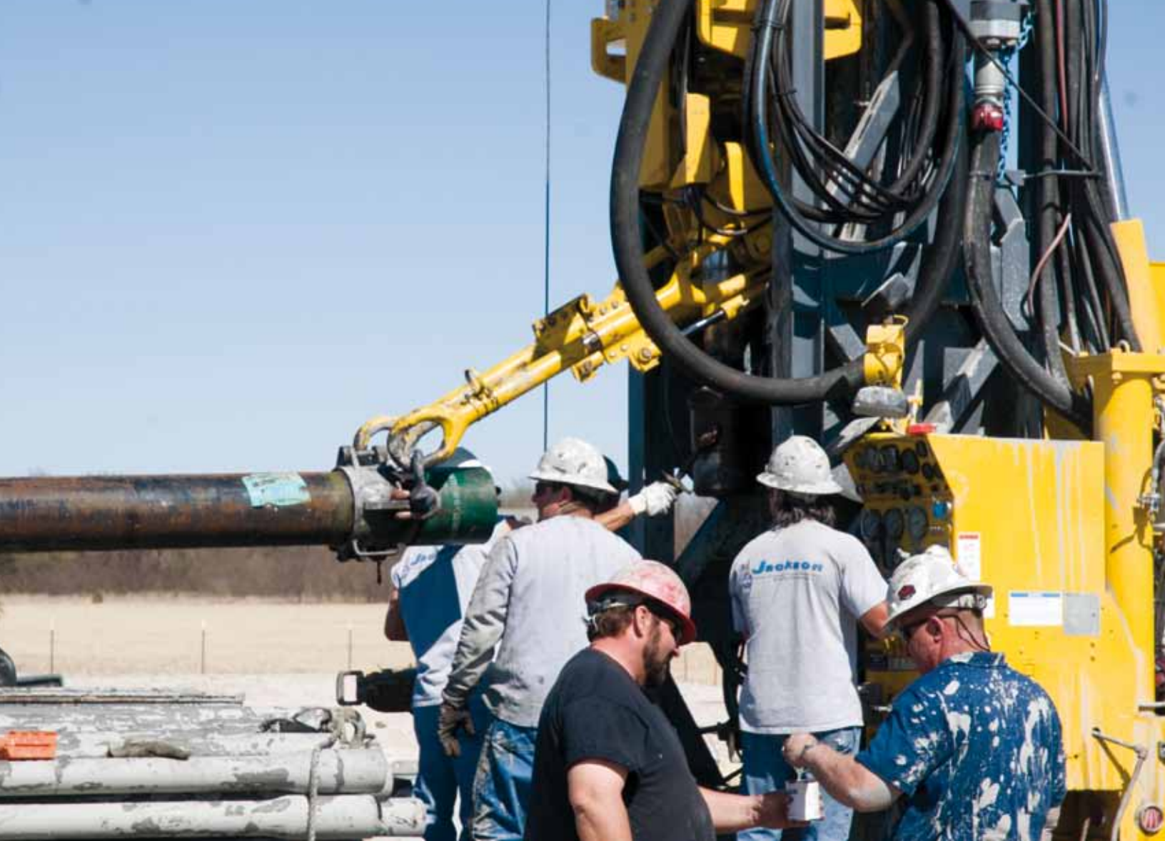
The RD20 XC handles this job's range 3 threaded 9 7/8-inch steel casing with ease.
