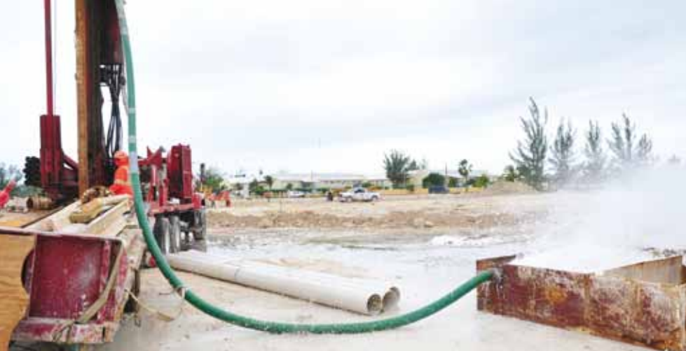
Cuttings from the discharge line are captured in a steel box so they can be hauled away or disposed of easily. Attaching the discharge line to the box anchors the line and diverts water away from the work area.
