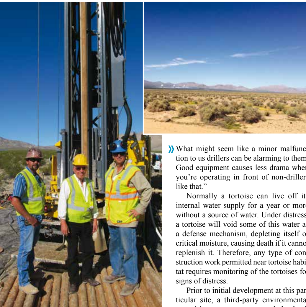
Miguel Chavez, AZCA owner Larry Siddall and Frank Chickey, Atlas Copco deep hole product support.
