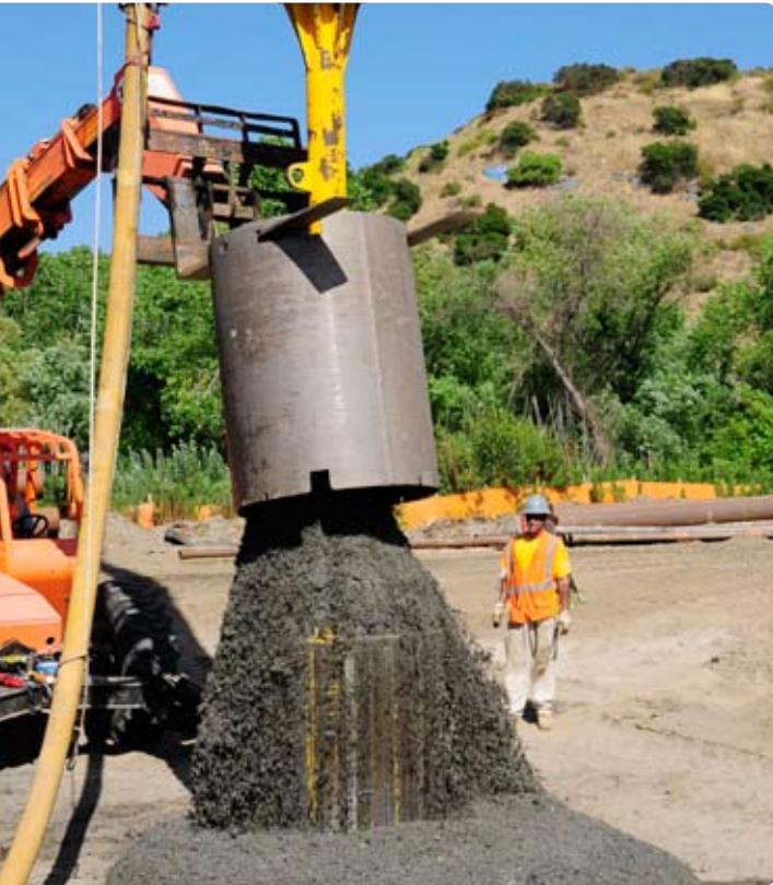
Cluster drills fitted with an assembly of DTH hammers are widely used in the USA for fast and easy drilling of large diameter holes. Above right, lowering a cluster unit into place and, at left, emptying the Calyx cuttings can.
