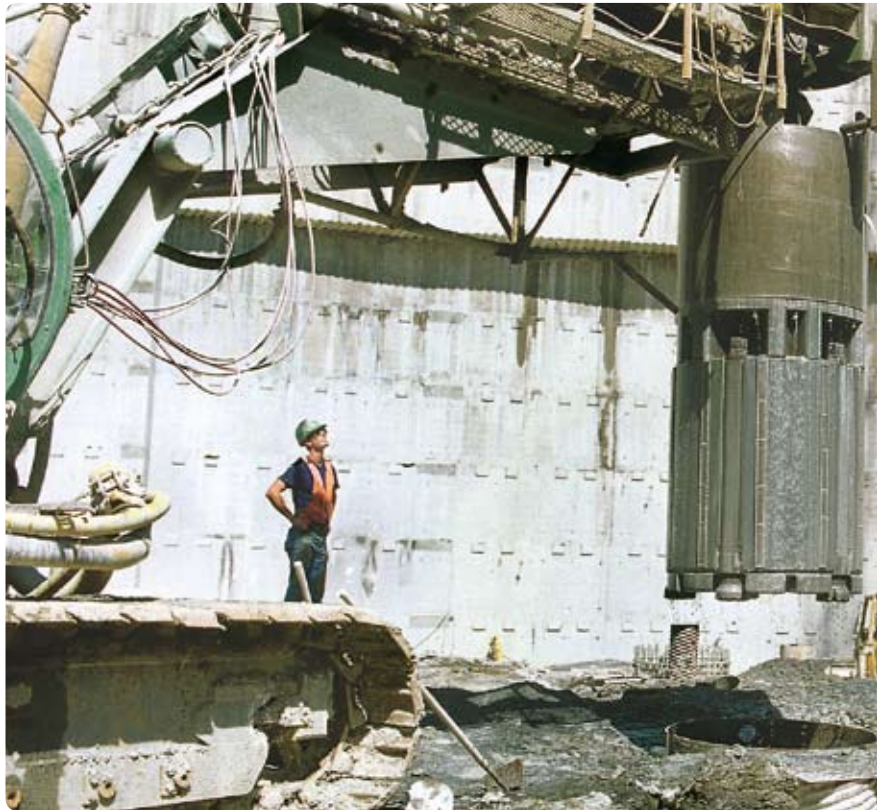
Cluster drills fitted with an assembly of DTH hammers are widely used in the USA for fast and easy drilling of large diameter holes. Above right, lowering a cluster unit into place and, at left, emptying the Calyx cuttings can.
