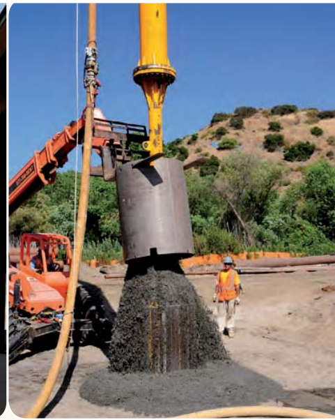
Cuttings are dumped from the Calyx basket, which collects cuttings during the drilling process.
