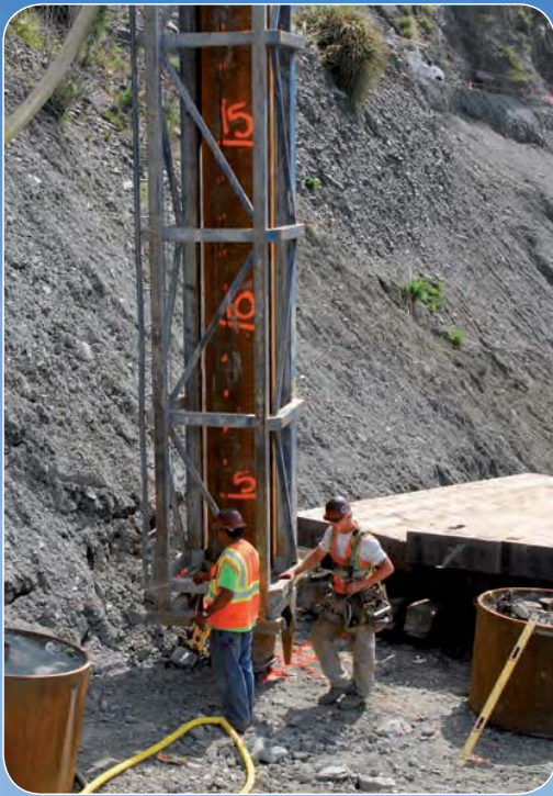
Workers check to see if the casing is plum.
