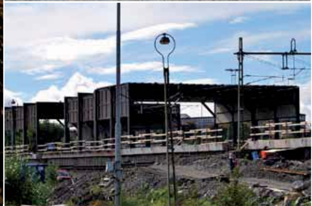
Drilling without disturbance: Above, engineers at work in the small hours; top right, Site Engineer Johan Blumfalk with the Elemex drilling system; far right, the shields that will protect the existing railway while a new railway bridge is built for the City Line trains.
