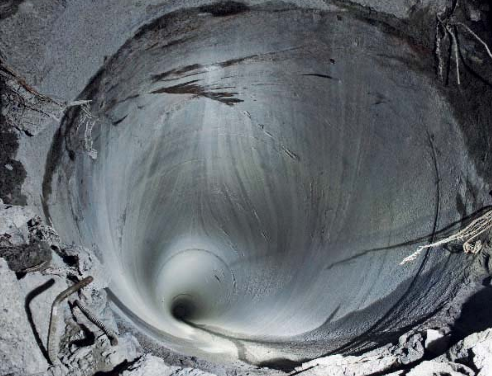
A prime example of fine raiseboring technology: Perfectly straight and smooth walls, bored at precisely the required diameter.
