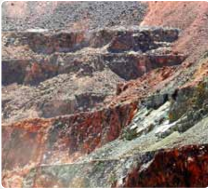
Typical sign: In mines where the drilling of the final slope is performed with drill rigs that are not suitable for presplit drilling the result is an unstable pit wall and benches that crumble and collapse over time.
