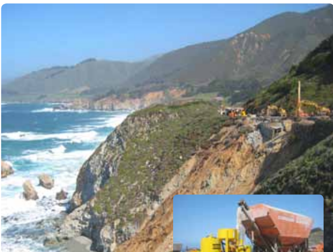
The Atlas Copco Unigrout system helping to stabilize the road in Big Sur.
