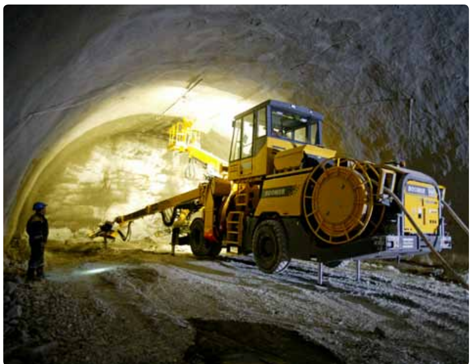
Olympic task: An Atlas Copco Boomer XE3C tunneling for contractor Bamtonnelstroy.
