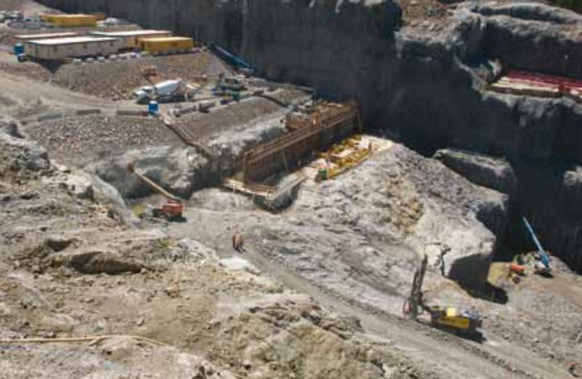
*To cut the wall in the background and for production work the company uses a ROC L8, such as the one seen here in the lower right corner. On unpredictable, pre-worked ledges such as this one overlooking the excavation, the company ties off a ROC D7, which can crawl down the steep grade as well as drill at a pronounced angle while the operator remains safely back from the ledge.*
