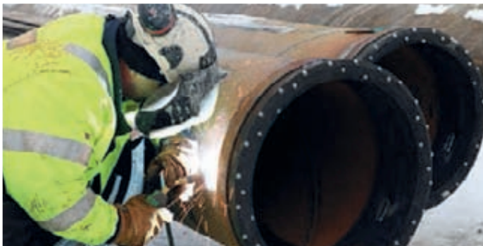
Clockwise from left: Welding the casing shoe with its oversize ring bit prior to drilling; aligning the interlocking casing wall; the retracted inner drillstring after pipe installation.
