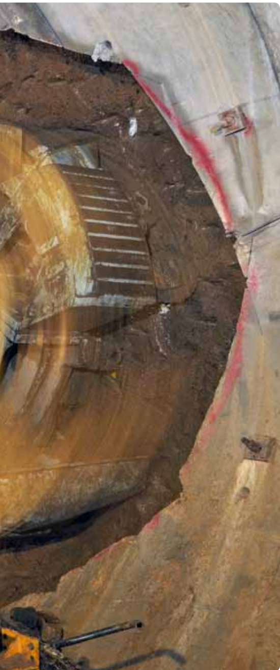
Drilling the pilot hole: A 311 mm hole is drilled in the tunnel wall where the relief duct is to be placed. On the opposite side, a reamer is attached to the drillstring and, pulling back to the raiseboring machine, the opening is reamed to a diameter of 3.5 m.
