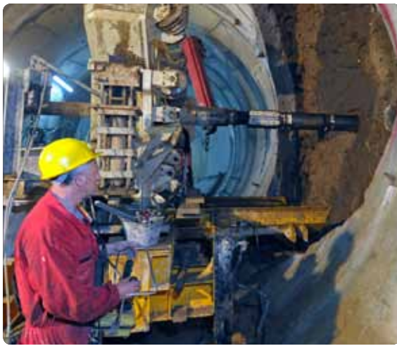
Drilling the pilot hole: A 311 mm hole is drilled in the tunnel wall where the relief duct is to be placed. On the opposite side, a reamer is attached to the drillstring and, pulling back to the raiseboring machine, the opening is reamed to a diameter of 3.5 m.
