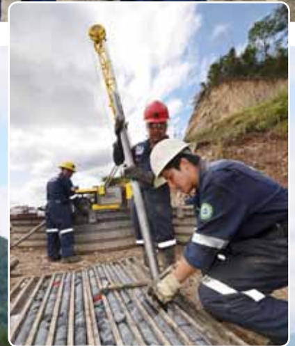
Core drilling in the beautiful Molango mountains with Atlas Copco drill rigs: Right, Carlos Cuellar holds the pipe while Pablo Guzman removes a core sample and places it into the box.
