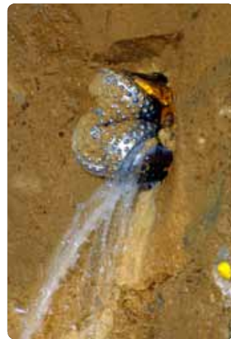
Drilling the pilot hole: A 311 mm hole is drilled in the tunnel wall where the relief duct is to be placed. On the opposite side, a reamer is attached to the drillstring and, pulling back to the raiseboring machine, the opening is reamed to a diameter of 3.5 m.
