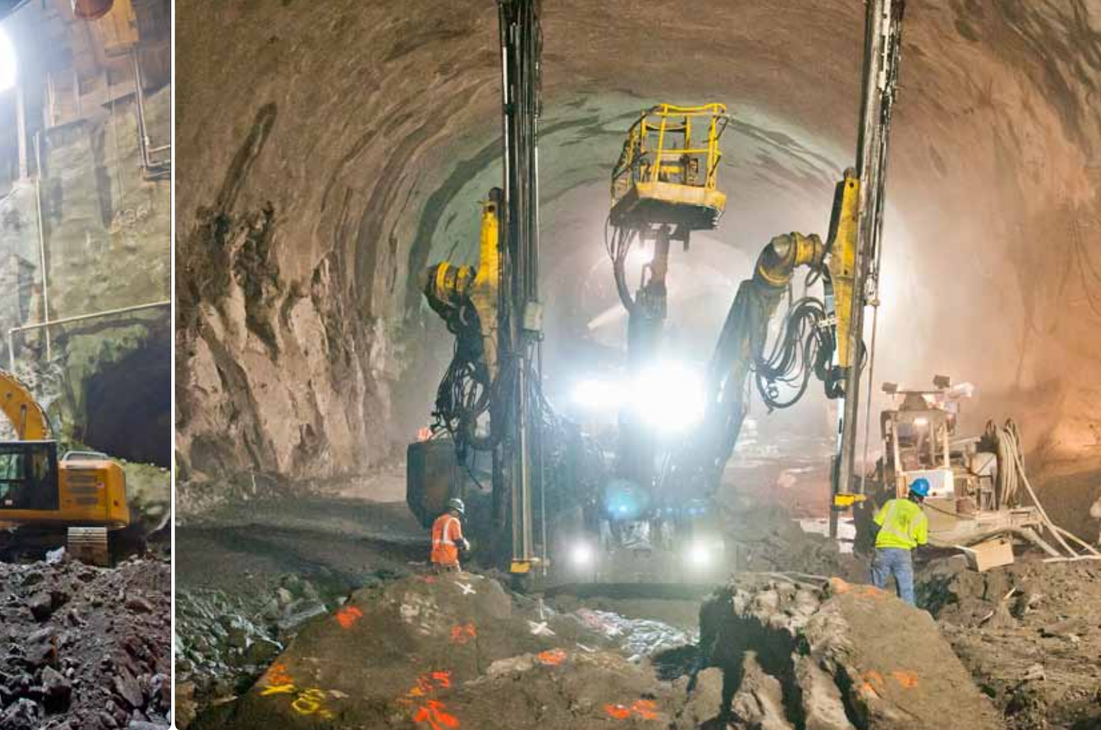
Benching the North Shaft: A Boomer T1 D had to be used to expand the lower level of the shaft to create sufficient space for the Boomer E2 C (above) to start vertical drilling.
