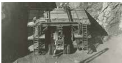
▲ One of two Atlas Copco PROMEC T 290 rigs, equipped with six TUNMEC R250 booms, is seen here in 1961 slashing one of the 11 penstock tunnels at Churchill Falls. The rig was raised on winches for blasting and lowered again to rapidly resume drilling. Mechanized long-hole drilling was introduced at this time with the Simba 22, significantly increasing drill meters per man hour.
