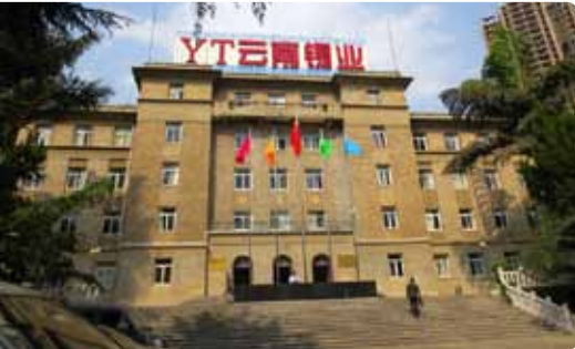
Big in tin: Headquarters of Yunnan Tin, the world's largest tin producer.
