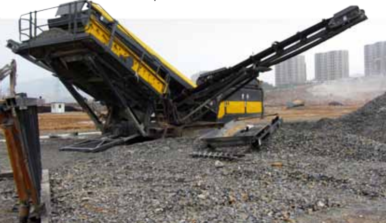
...material screening with the compact HCS 3715 mobile screener...
