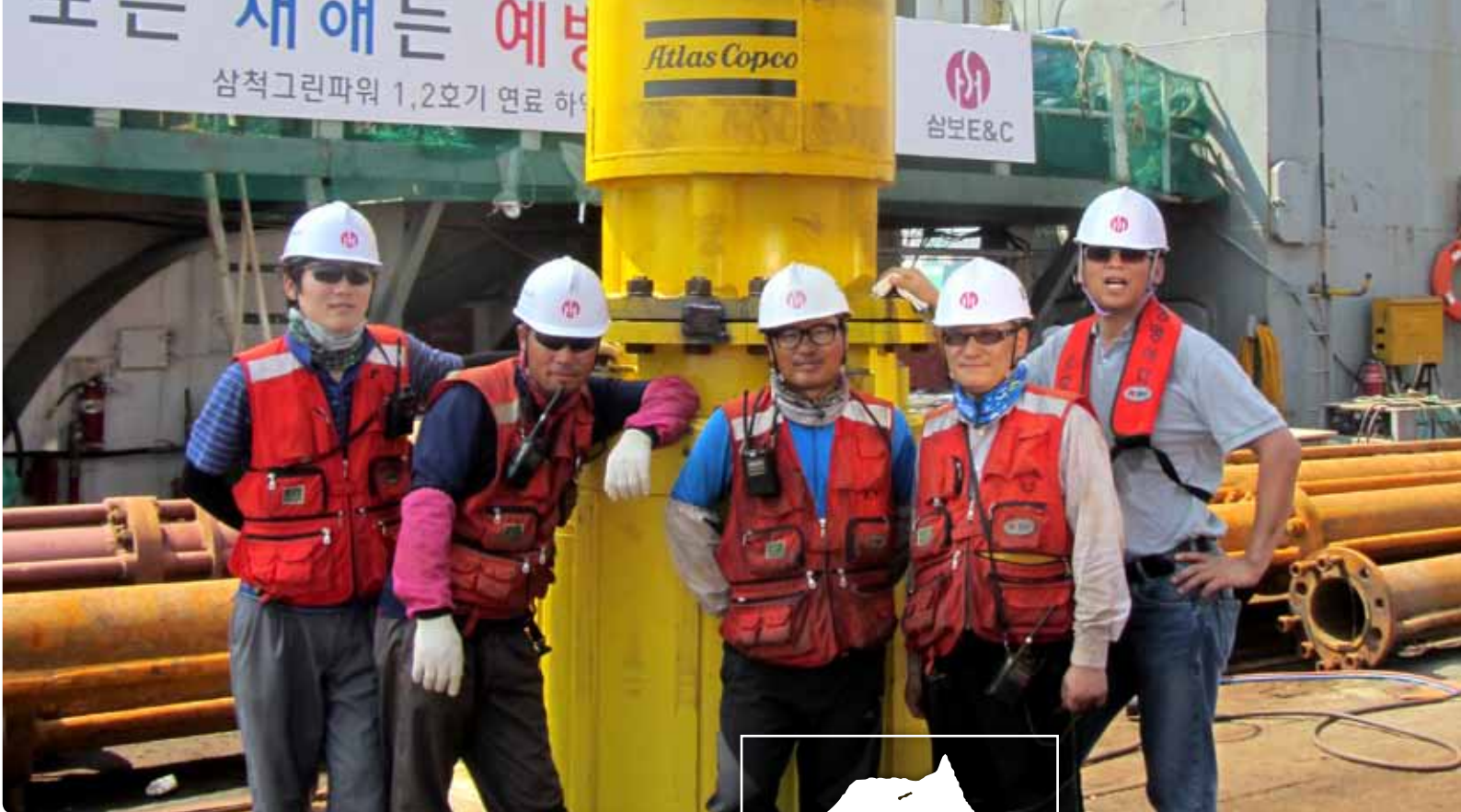
Left, the Atlas Copco cluster drill is lowered into the rig. Above, the proud Korean drill crew at Sambo E&C.
