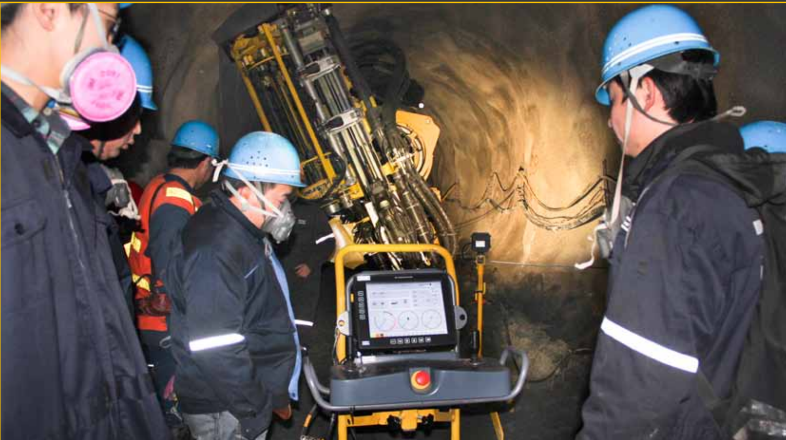
Under ground: Setting up for the first demonstration of the Simba M4 C rig's many capabilities.
