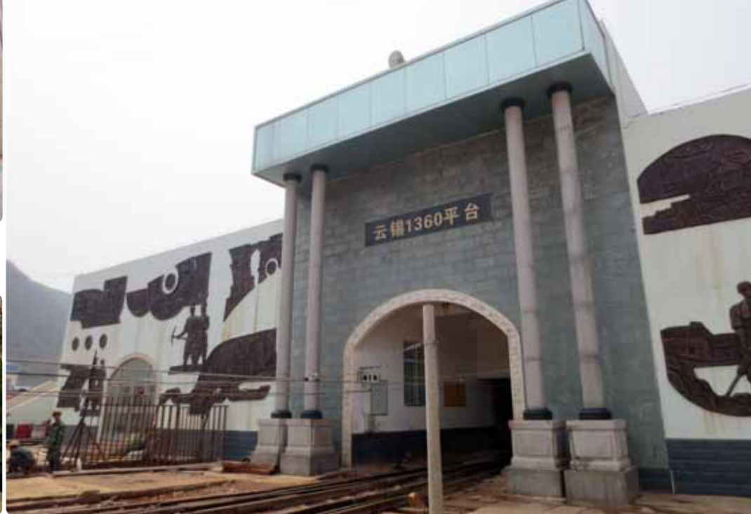
Profitable solution: Entrance to Song Mine in Yunnan province where the Atlas Copco equipment helps to produce more than 1.3 Mt of tin per year.
