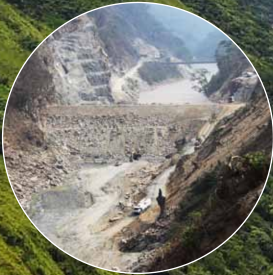
Constructing the dam at Ituango.
