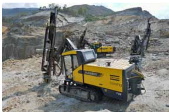
On the surface: FlexiROCT35 rigs work both above and below ground.
