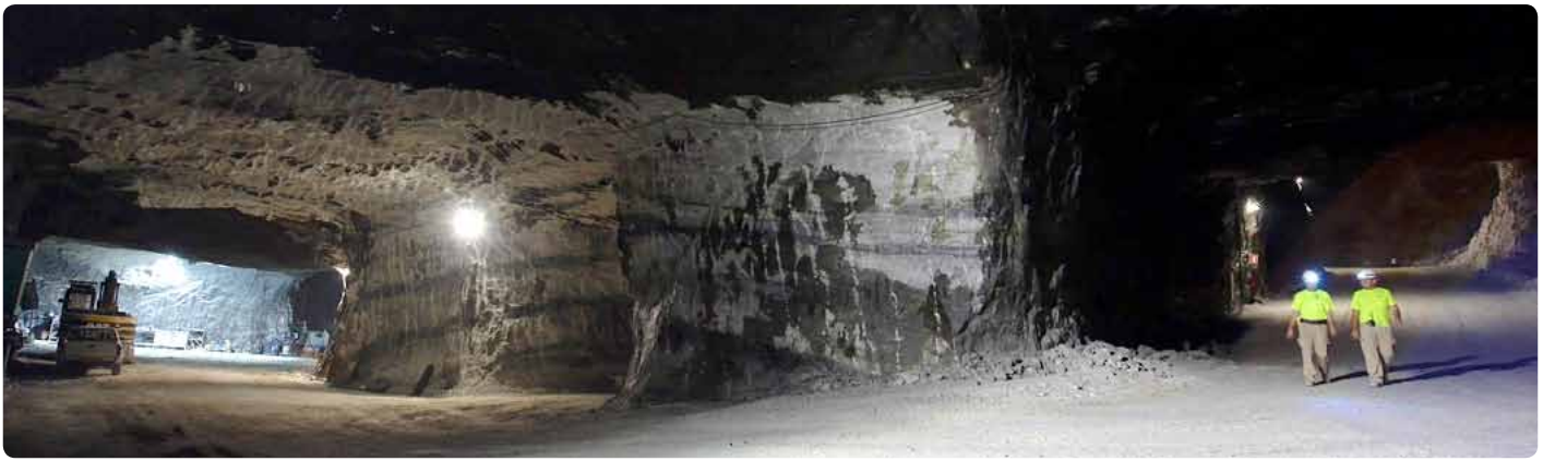
Strength and reliability: The underground Xauxa marble mine in Barcelona, Spain, has carried out a new rock reinforcement program based on Atlas Copco's Swellex Spartan rock bolts.
