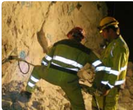
Good pull: Tests with the Swellex Spartan showed a bolt elongation of 6%.
