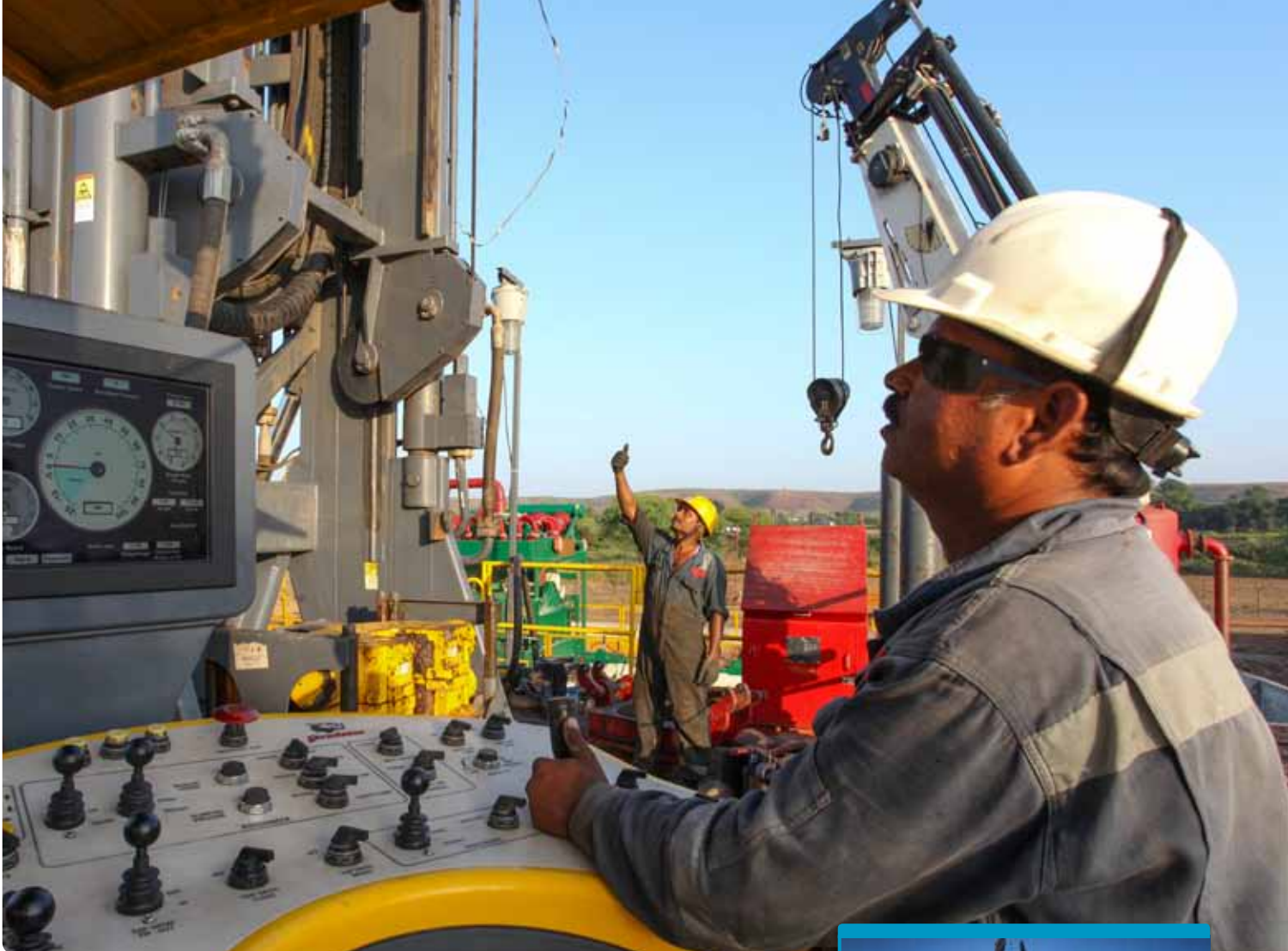
Manning the control panel: The Predator completed the targeted depth of more than 2 000 meters on time and with a “best performance per shift” which the company believes is a record in the Indian O&G industry.
