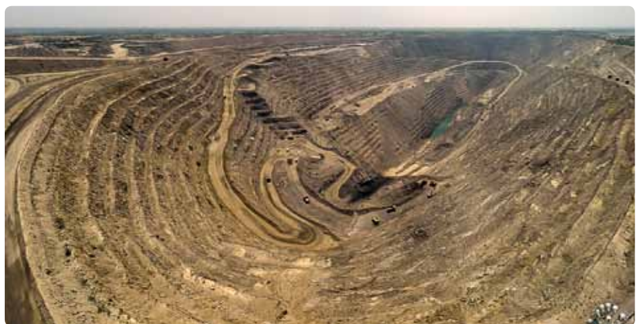
Going underground: Below the 372 m level, excavation of the Rampura Agucha orebody continues underground with proven and probable reserves estimated at 100 million tonnes, will have a lifespan of 25 years.
