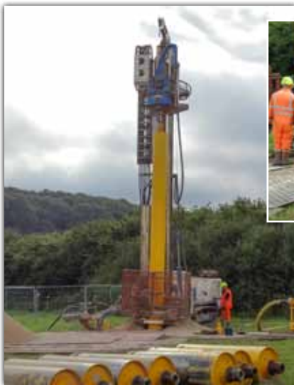
A new water well for the soft drinks industry: Successfully completed with Atlas Copco's QL 120 hammer.
