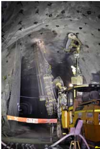
The trial begins: The Boltec MC in the El Teniente mine.
