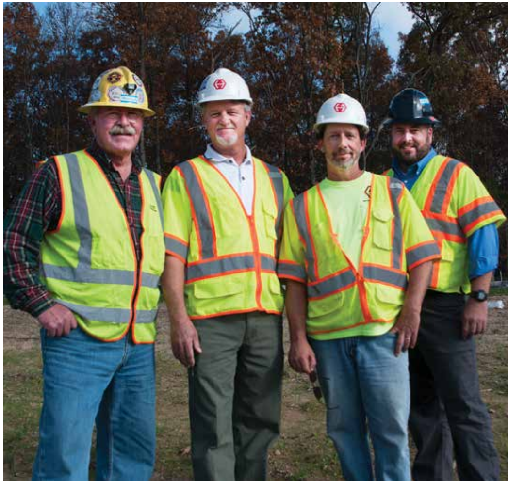
This area undergoing site prep will be all houses soon. Shown are Craig Mooney (territory manager for Atlas Copco), Tom Ashbaugh (Hazel blasting superintendent), Ricky Clatterbuck (Hazel blasting assistant superintendent), John Swift (Atlas Copco—Abingdon manager).
