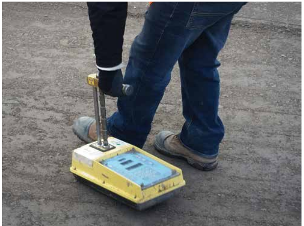
Compaction testing confirms the LG500's effectiveness.
