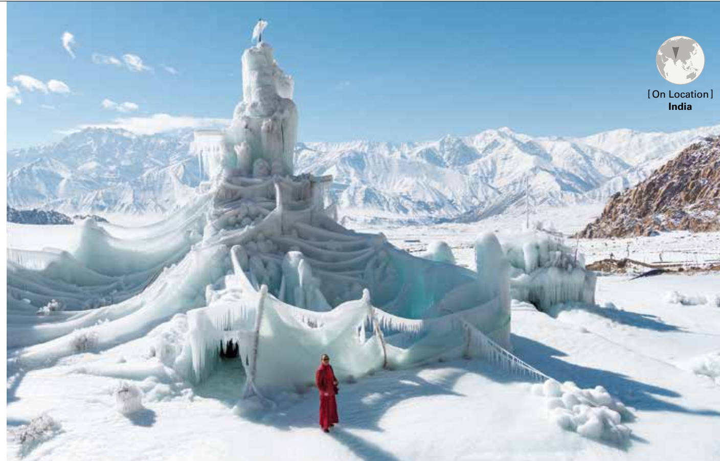
Engineer Sonam Wangchuk is the man behind the idea of the ice stupas. His invention has helped villagers in Ladakh to store winter water to use in springtime.
