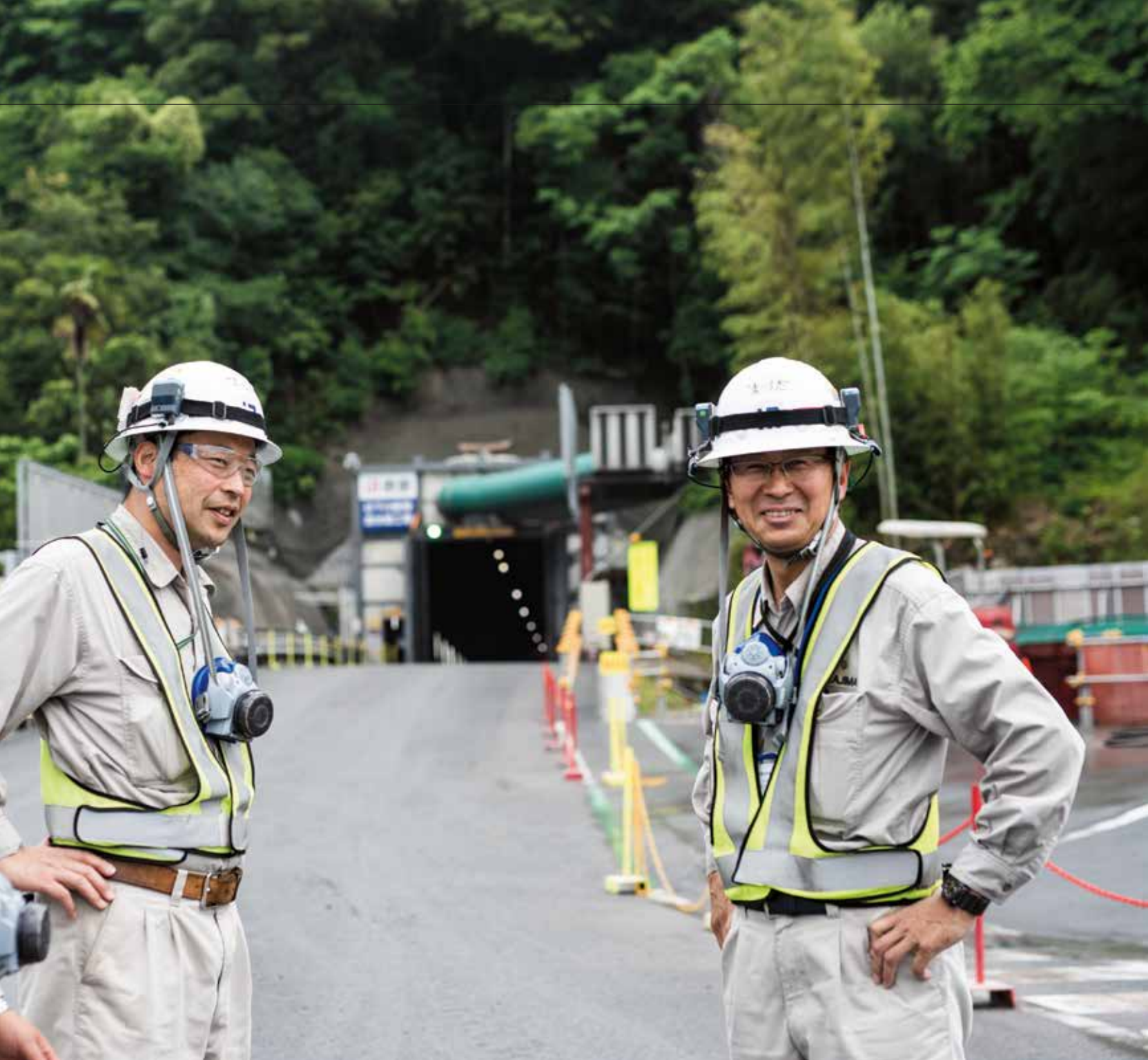
Experienced Kajima Construction superintendents ready to supervise the work at the Kusakagawa New River Tunnel project.
